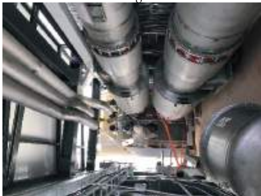
Figure B.1.9: Installation of warmlines and Group-X cryolines on cryo-bridge.
