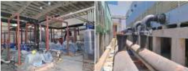
Figure A.6.1: Ongoing installation activities.
