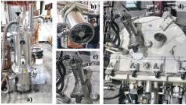
Figure A.4.11: a) Pump test setup with AVS dome, b) lifting pump for integration to HHF, c) showing mounted pump and the gate valve, and d) top view of HHF chamber with integrated pump.
