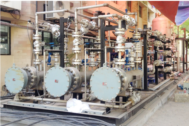
Figure A.2.3. High Pressure High Temperature Water Circulation System (HPHT-WCS) for HHFTF
