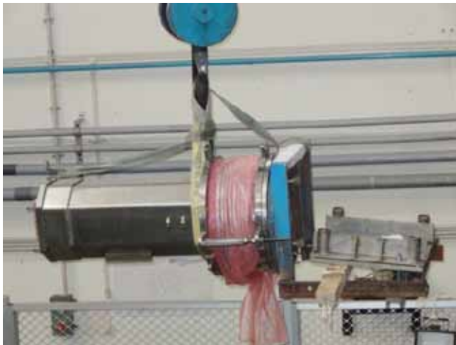
Figure A.1.2.4 The In-vessel module is lifted and inserted into the radial port using special lifting device with counter weight to balance the non-uniform load of IVM and avoid interference with vertical coils.
