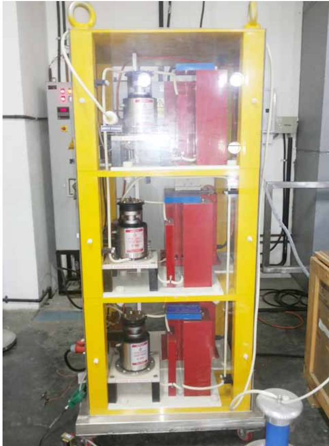
Figure B.2.5. Ignitron based crowbar protection system
