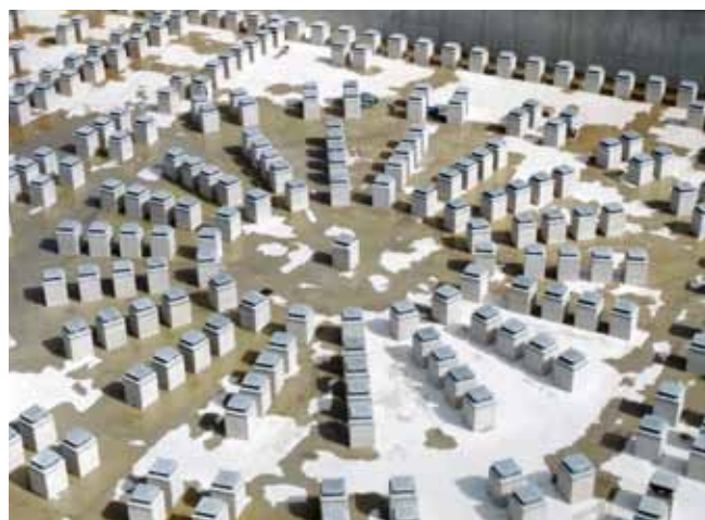
Figure B.2.2.2 The tokamak building foundation
