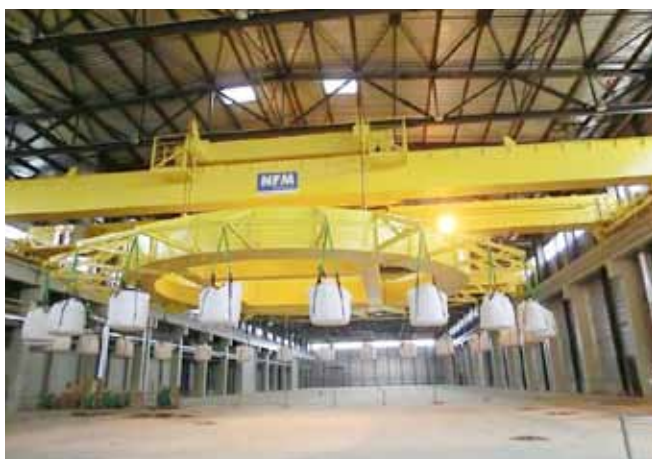
Figure B.2.2.3 Poloidal Field coil winding building
