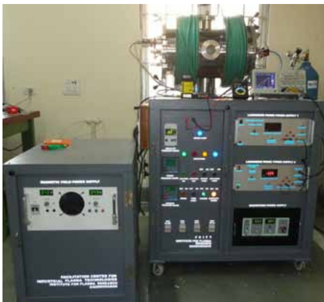
Figure B.1.1.1: Photographs of the CDPS system installed at Delhi University
