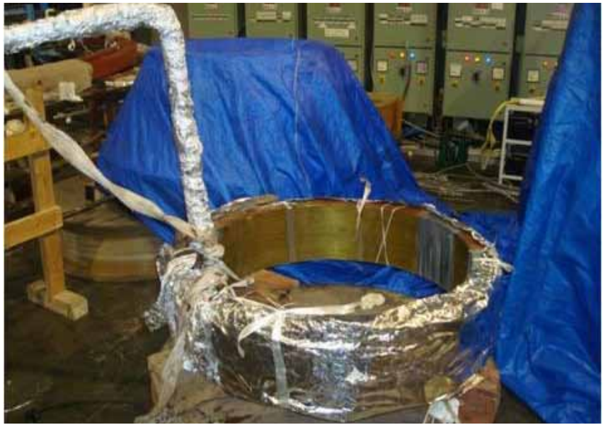
Figure A.1.2.1.3 Successful refurbishment of PF-2 top coil
